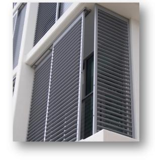
Aluminum louver window is a casement window without glass but with horizontal slats instead. The slats are angled to admit light and air, but to keep out rain and direct sunshine. The slats are made of aluminum and the angle of them can be adjustable or fixed.
