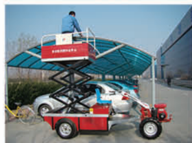
Building and fixing shed
