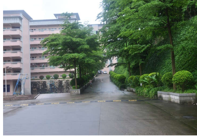
Corner of industrial park
