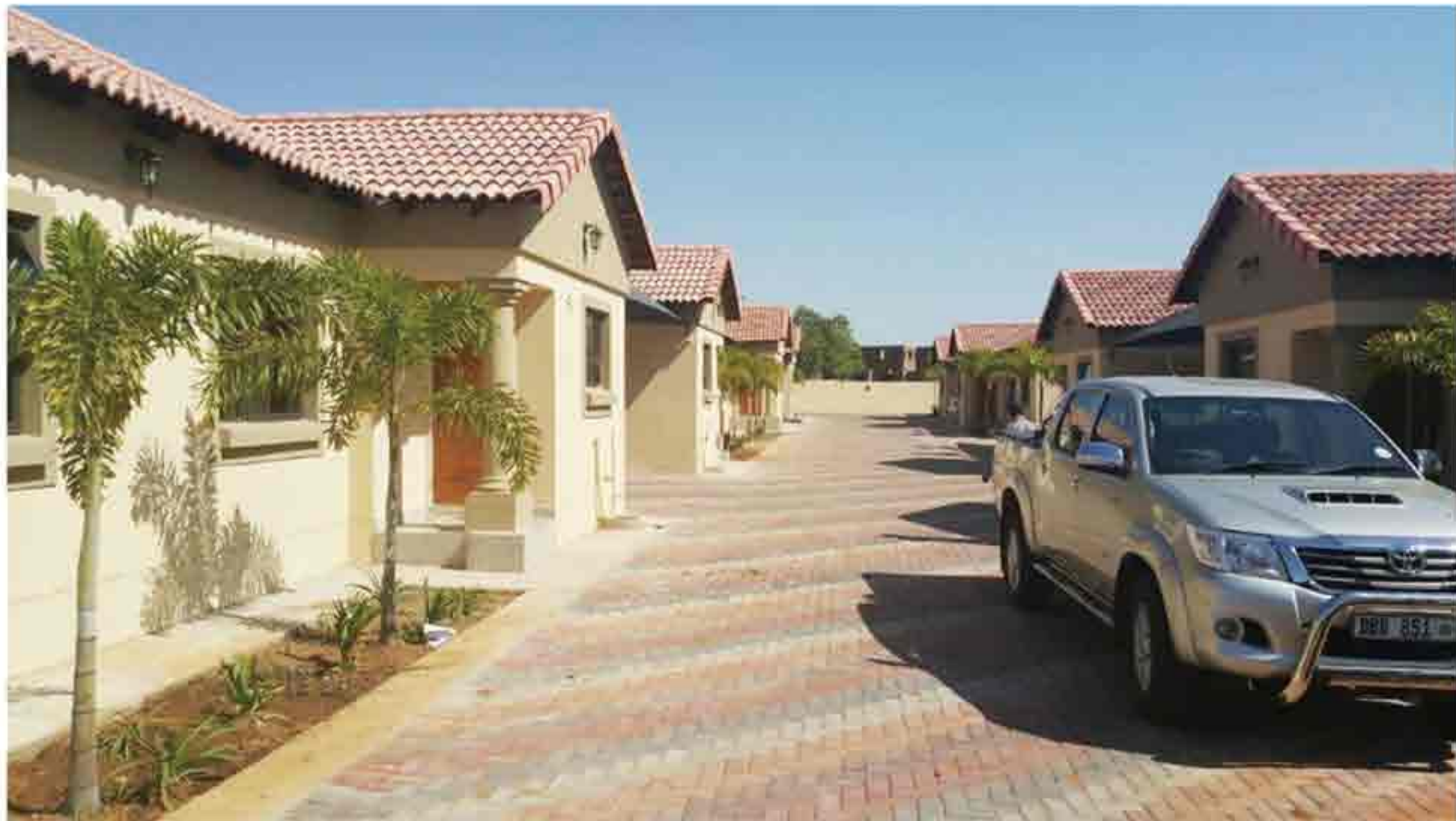
▲ South Africa Project
